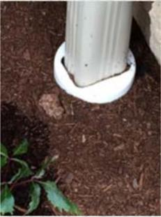
**Above ground surface water and roof water around the perimeter of the HOME needs to be managed properly. You as a BUILDER will have to educate the new homeowner, if not structural damage can occur!**
