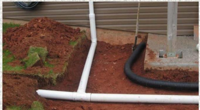
greater) to divert water away from the foundation or pier is a must... Other areas of concern such as roof gutter drain spouts should always be properly piped & diverted to prevent the soil adjacent to them from saturating in the fall and causing FROST HEAVE next to the foundation and/or pier.
