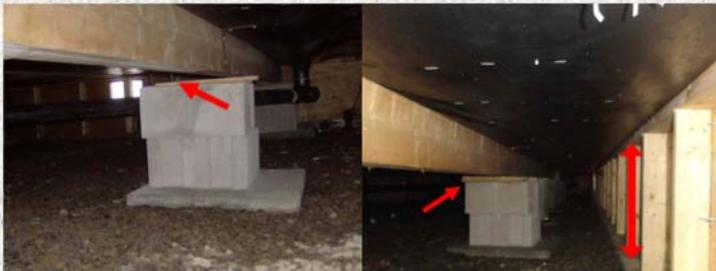
B) The skirting is not acting as a structure but because the siding panels are in direct contact with the ground they are deflecting when the ground freezes. Result: Unattractive bows and cracks in the siding panels.
