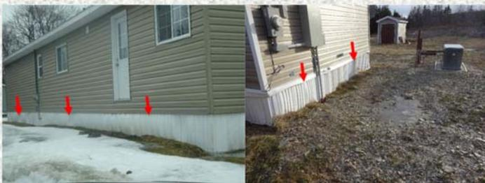
There are several options in preventing the above mentioned. The rule is to allow for clearance of approx. 2” (50mm) to prevent frozen ground from lifting either the siding or the framing of the skirting.
